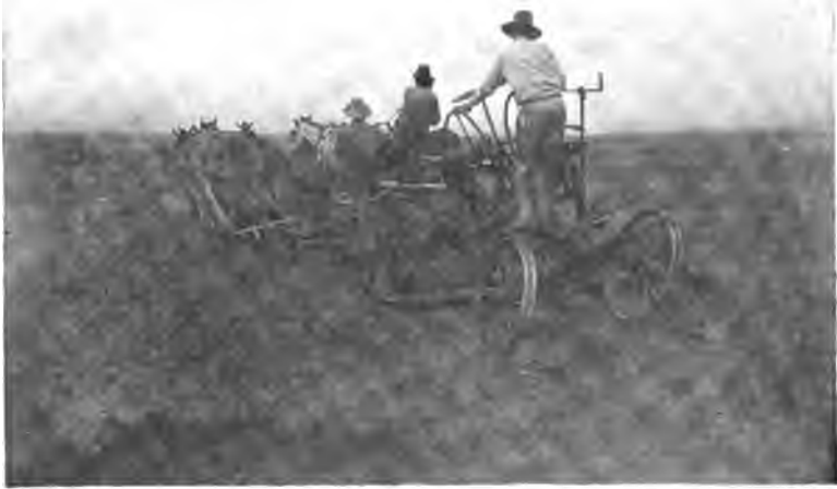
FIG. 74.—Building Lateral in Montana with Ditching Machine.
